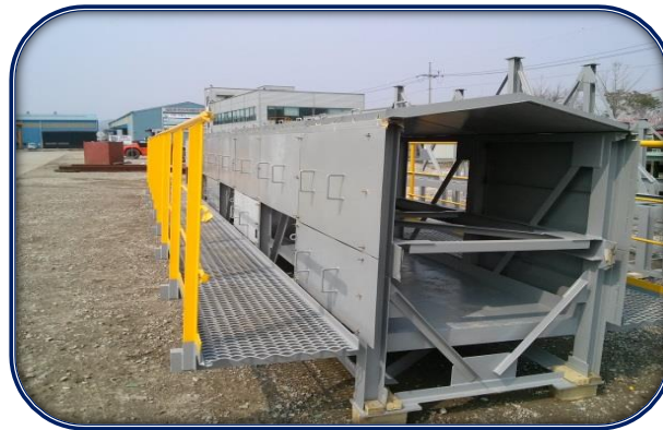
광양POSCO SNNC BELT CONVEYOR WARKWAY포함전체조립납품
