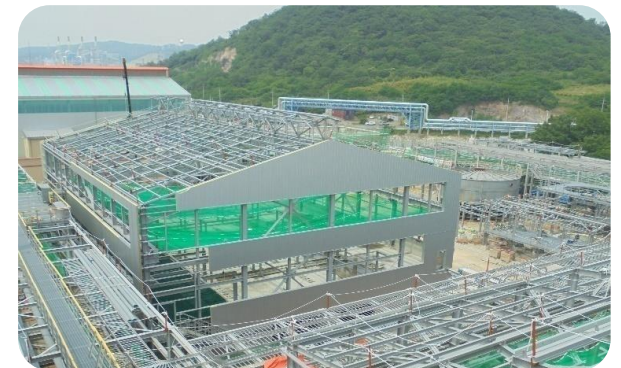
GS Caltex BIOBUTANOL DEMO PLANT Project
